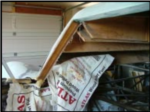
Picture 1, Caption: Work on the door jambs includes building flanges to mount seals around window frames. Fiberglass with a thickening agent (Cab-O-Sil) is used for lay up on this vertical surface.
